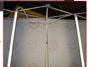
Link cable connection close up.
