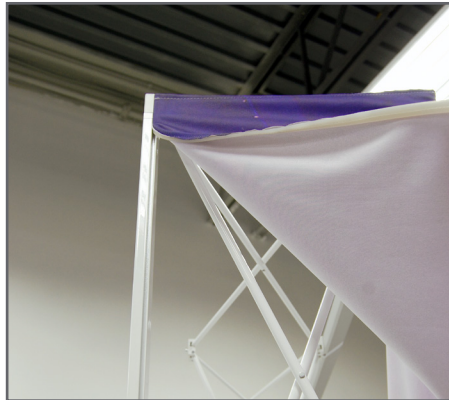
4. Install front graphic, start with endcaps
