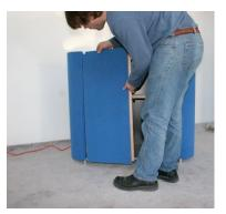
8. Install the doors with the longer pin up. Locate the holes in the frame and insert the longer pin into hole in the underside of the top frame and then drop in into the hole in the bottom frame.
